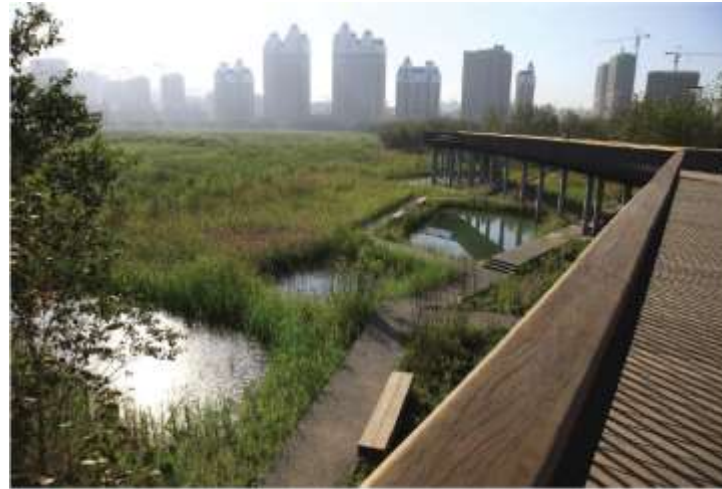
QUNLI STORMWATER - CHINE
